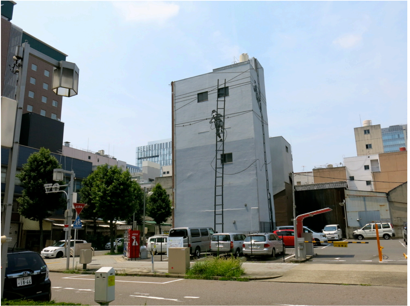
Wall painting on the former Tamaya building by Portuguese artist Rigo 23 who was inspired by a 1952 photograph of Nagoya workers perched on ladders. Choja-machi site.
