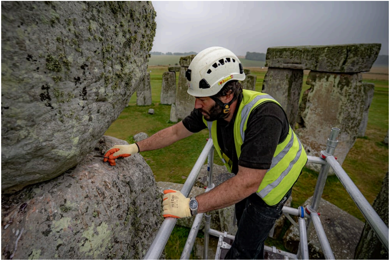
Conservator James Preston uses a pointing spoon atop scaffold erected inside the stone circle at Stonehenge. Photo: Ben Birchall/PA Images via Getty Images.
